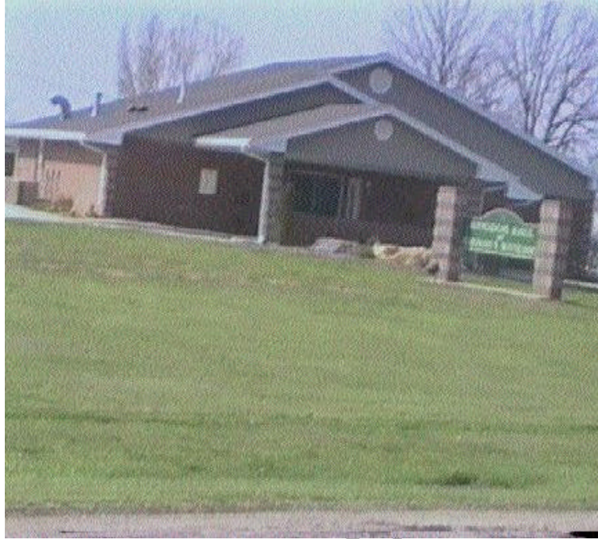
Photograph courtesy of H. Stone
